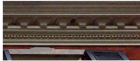
Denticulated and modillioned wood cornice
